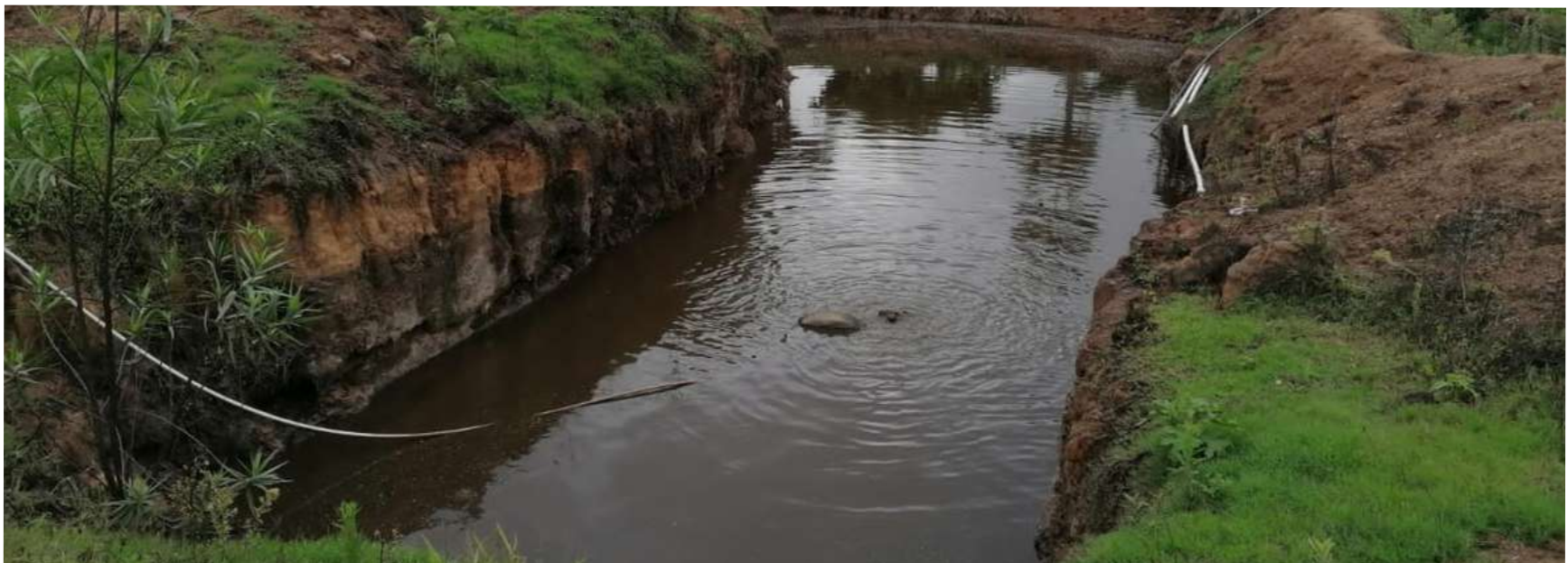
Installing an air bubbling system in a wastewater treatment pond
